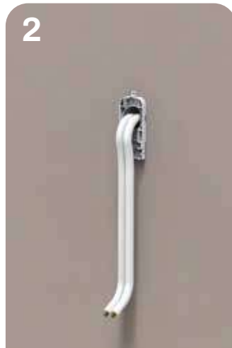
2 Insert the refrigeration lines and the power cable into the wall hole
