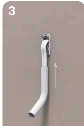
3 Place the refrigeration pipes and the power supply in the corrugated protection pipe
